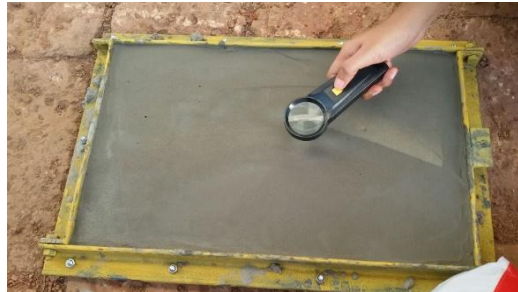
Observation of cracks
