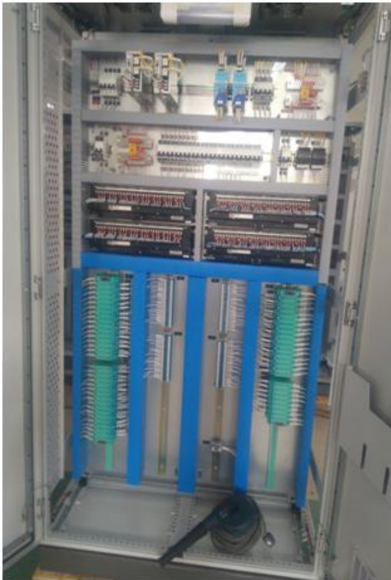
Figure 5: Power Distribution Panel
