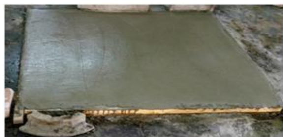
Fig. 7.6 Finished layer of slab
