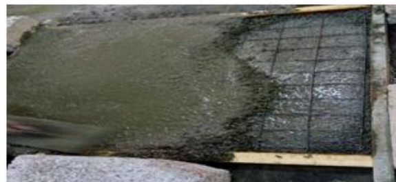
Fig. 7.5 Concreting of slab
