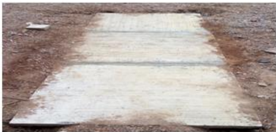
Fig.7.7 Completed pavement surface
