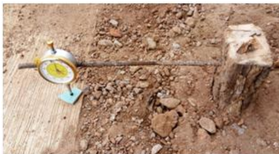
Fig. 7.8 Dial gauge fixed to slab
