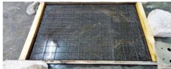
Fig. 7.4 Placing of skeleton mesh in mould
