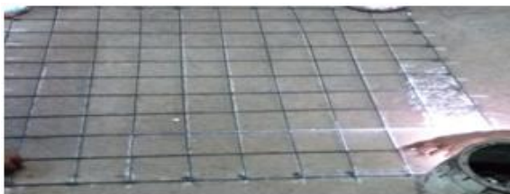
Fig. 7.1 Welding of skeleton structure
