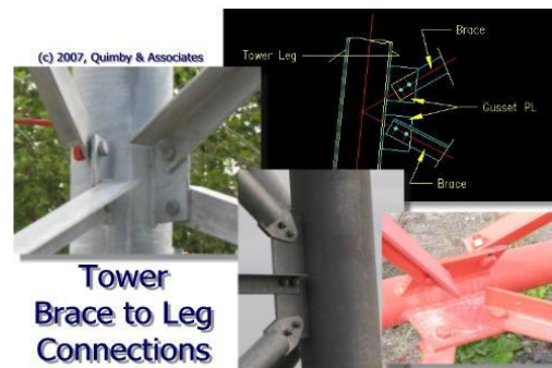
Figure 3: Tower Brace to Leg Connections
