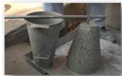
Fig -12: Slump Test in Progress
