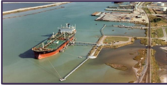
Fig. 1 Reinforced concrete LNG Terminal over View (source: www.marineinsight.com)
