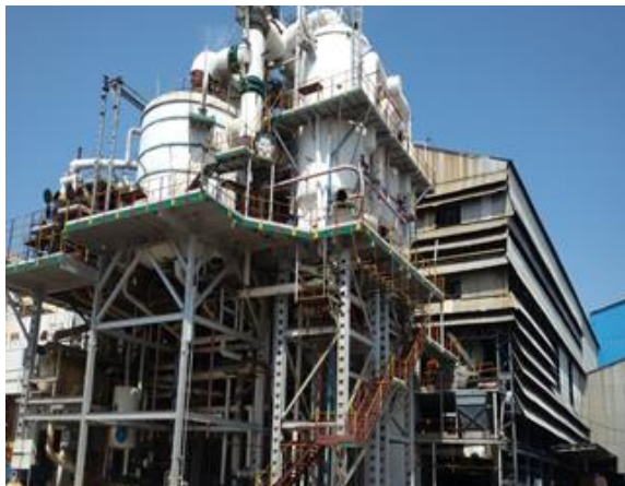
Fig 3.1: Site view of KCP sugarcane factory at vuyyuru, Andhra Pradesh
