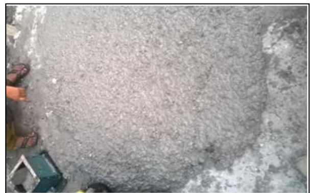
Figure 1. Mixing of geopolymer concrete
