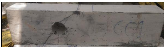
Fig. 7. Crack pattern of Control beam with opening CO1
