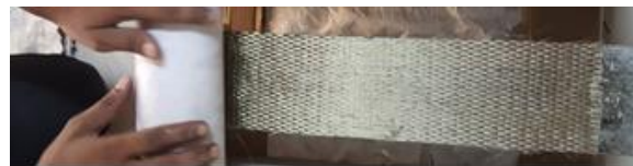
Fig. 6 Application of BFRP sheet
