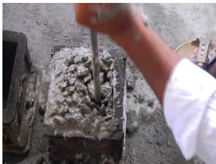
Fig -5: Casting of cube moulds
