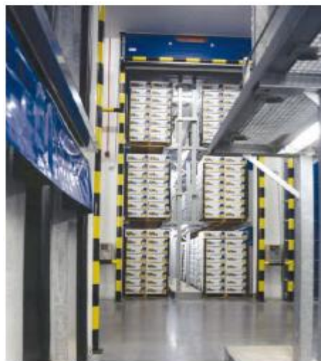
Side curtains with reversible airflow[10]
